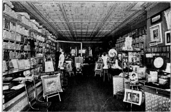
INTERIOR, GOODMAN PAINT AND WALL PAPER CO'S STORE
